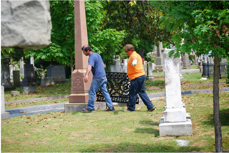
Unloading one of numerous sections of the restored Palmer Fence.
