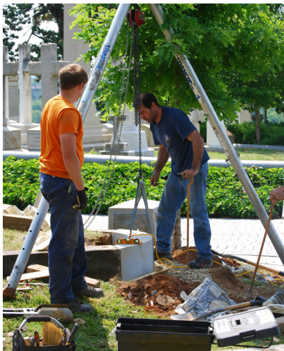
Workers placing a curved granite foundation for the Palmer Fence.
